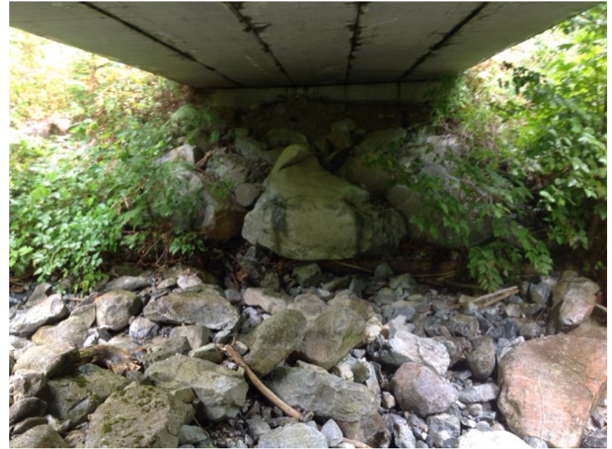
Left Bank Abutment when facing downstream
