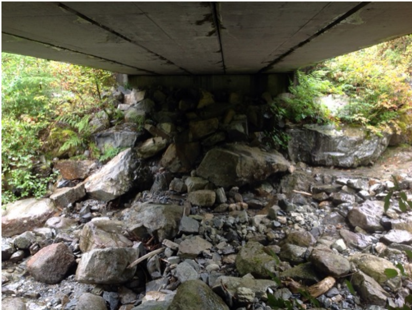
Right Bank Abutment when facing downstream
